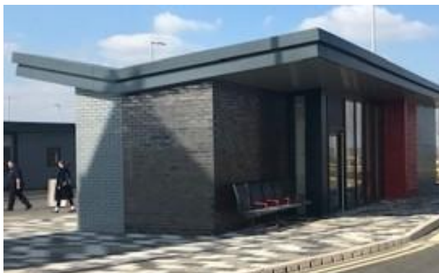
Figure 2-2: EMG1 Bus Interchange
